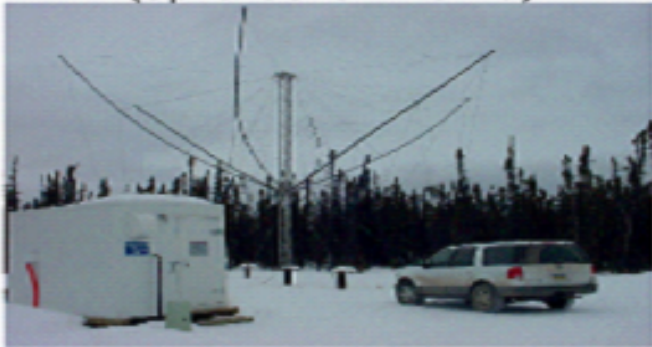
HF Receiving Station (Spira-Cone Antenna)
